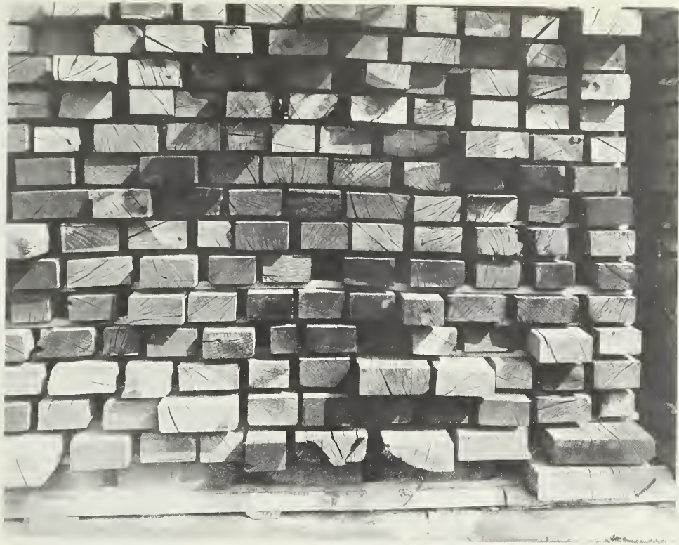
Figure 40. --End checking and splitting in heavy oak.
